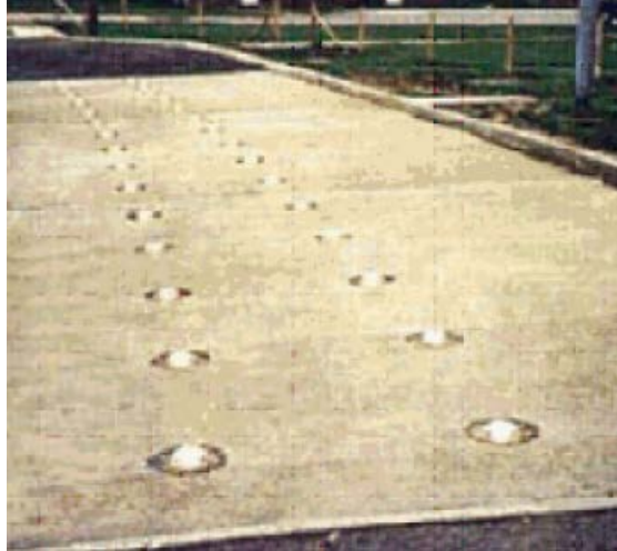
Figure 2.6. In-pavement warning lights for wrong-way vehicle (Cooner, Cothron, and Ranft 2004).
