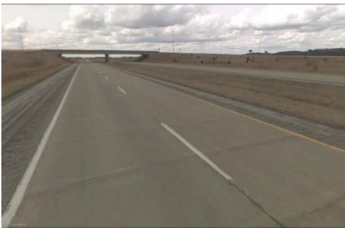
Street view of wrong-way crash site (Data Source: Google Maps)
